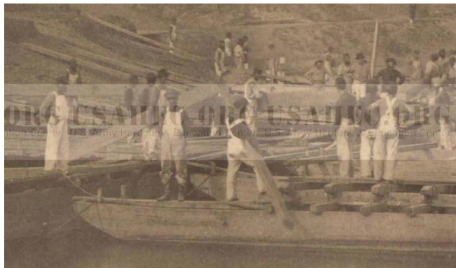
FIG. 10. Engineers wearing their authorized white canvas overalls are seen here assembling a pontoon bridge across the east branch of the Potomac River near Washington, D.C. in September 1863. (AHEC)
