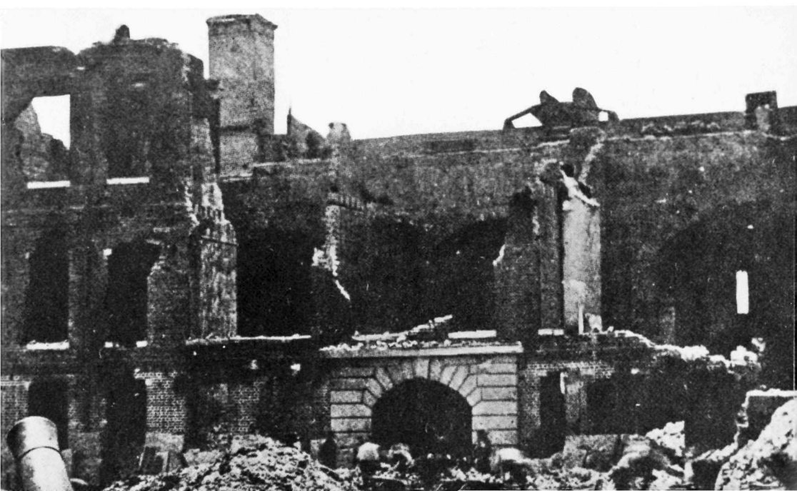
Interior of the Gorge after the April 1861 bombardment. Parade entrance to sally port is at center.
